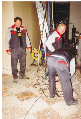
Installation of monitoring-lines
