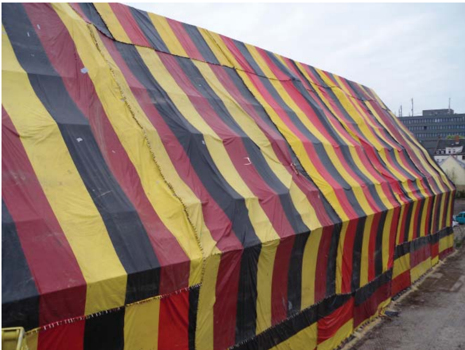
Fig. 1 - Tarping of a woodborer-infested structure (40000 m 3 ) using a form fitting tarpaulin.
