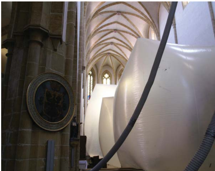
Fig. 3 - Air inflated balloons help to save Vikane fumigant.
