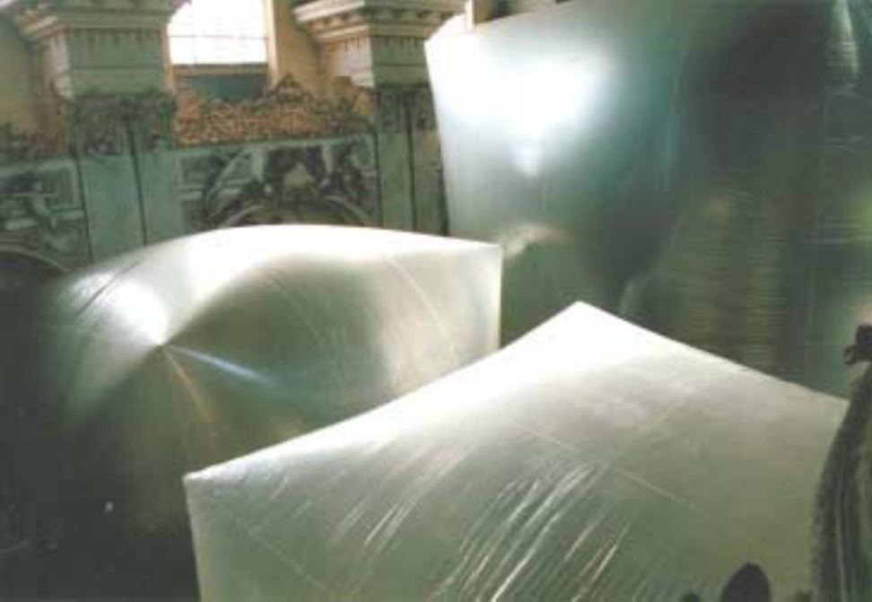
Fig. 5 Air inflated balloons help to save Vikane fumigant
