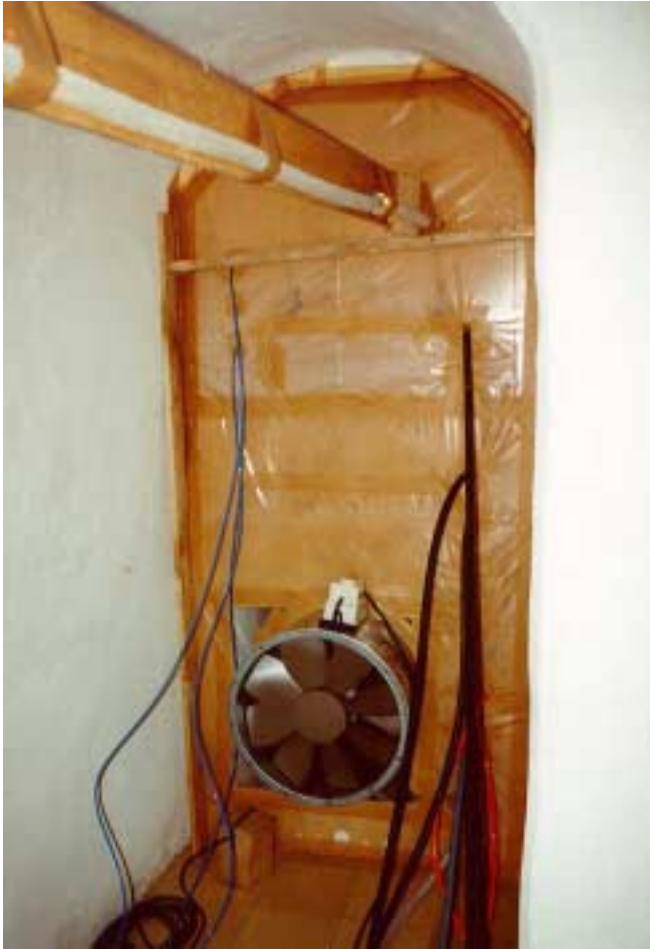
Fig. 4 Set up for the Pressure Test of a church
