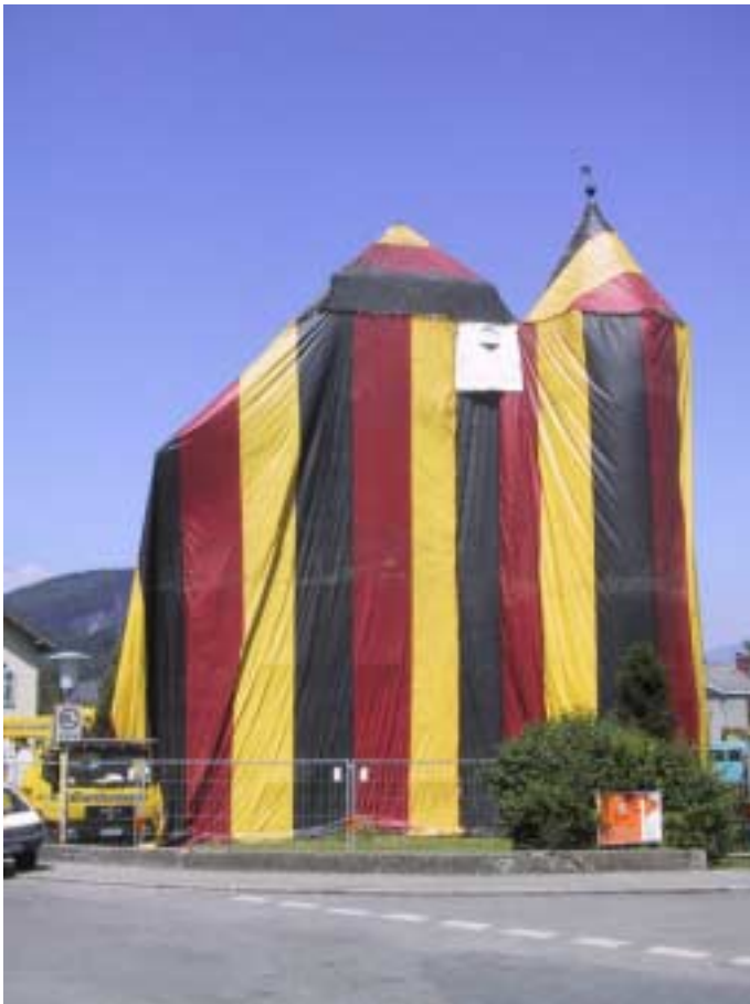
Fig. 2 Tarping of a woodborer-infested castle using a form fitting tarpaulin
